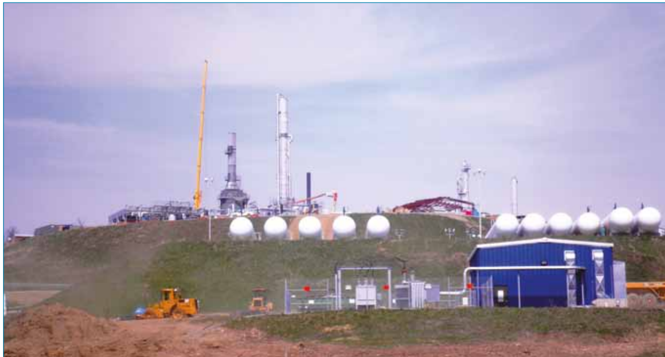
Gas processing plant near Houston, Pennsylvania
